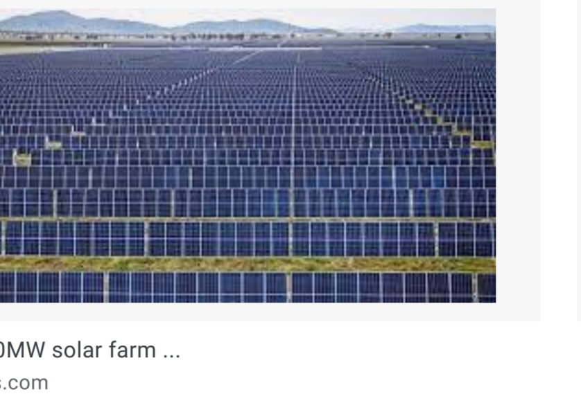
stepwise 500MW solar farm ... rechargenews.com
